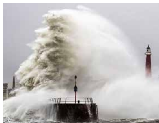
Figure 2 - Wave overtopping event at a coastal structure, see also Van Gent et al. (2023).
